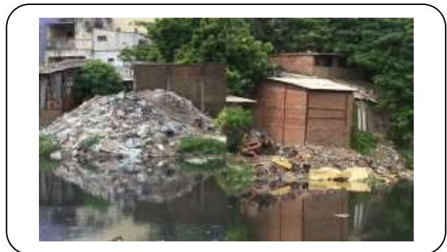
Fig. 9: Illegal dumping of materials in the river.
